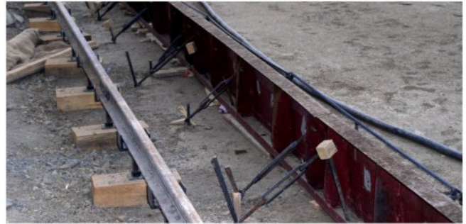
SIDE SHUTTERING ARRANGEMENT
