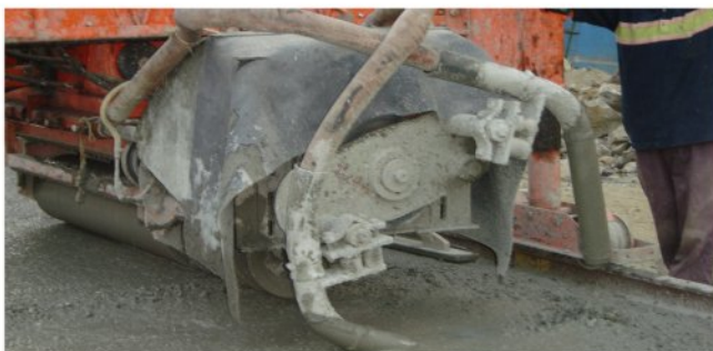
NEEDLE VIBRATOR ARRANGEMENT
