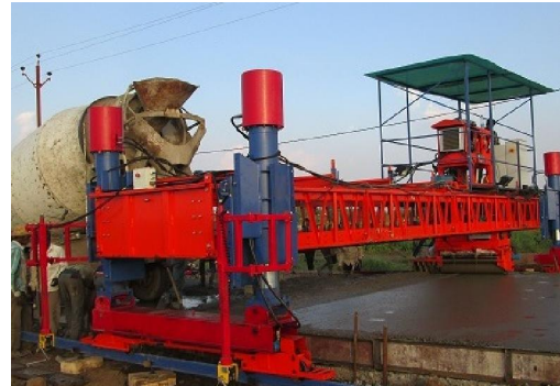
HYDRAULIC DRIVEN BOGIE
